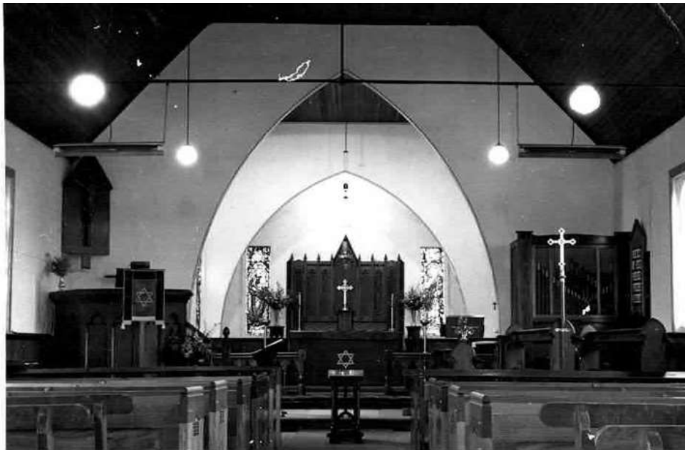
The nave and sanctuary of the original church.
